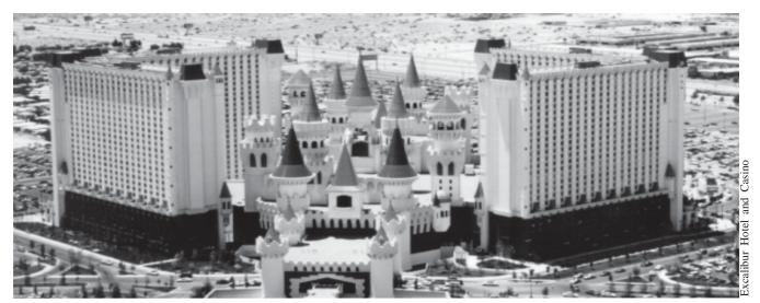
Figure 1-The four towers of the 28-story Excalibur Hotel in Las Vegas are load-bearing masonry.
